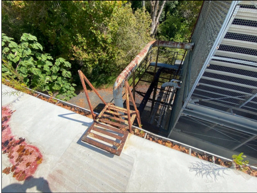
81 - View of upper roof ladder
