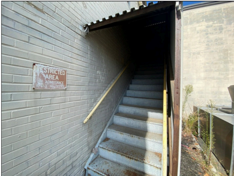
120 - Fire stairs at east side
