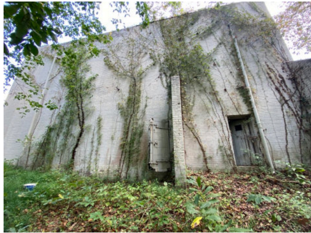
West elevation (note ivy on walls)
