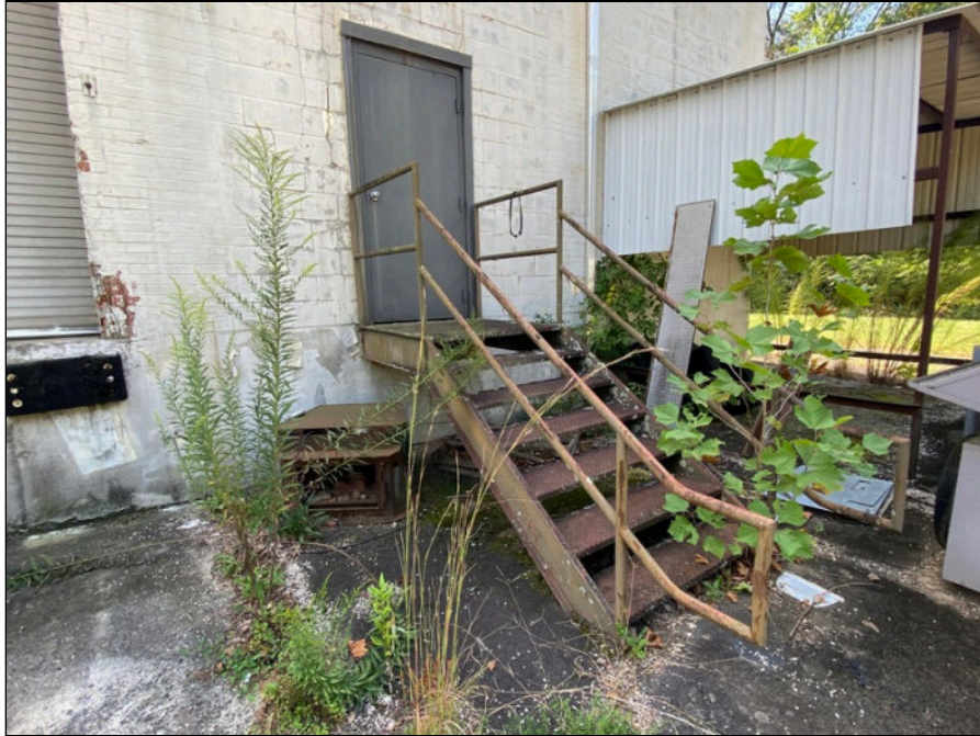
47 - Metal steps at doorway
