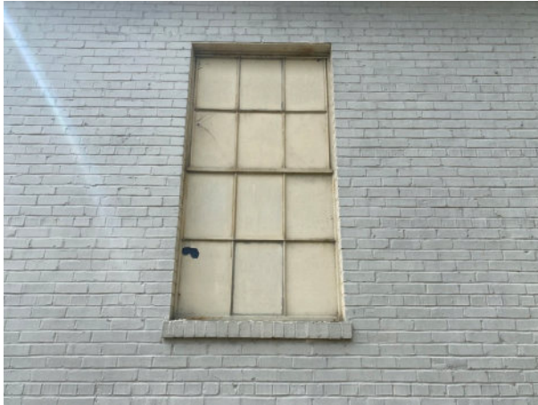
Typical steel window (exterior view)
