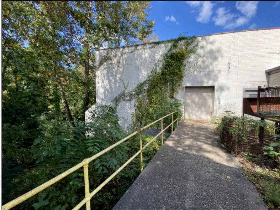
27 - Walkway at west side
