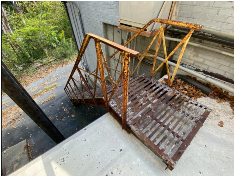
80 - View of lower roof ladder
