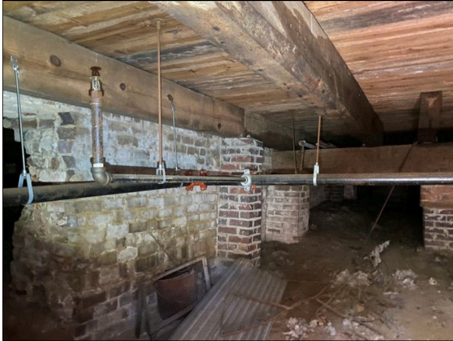
39 - Crawlspace below floor
