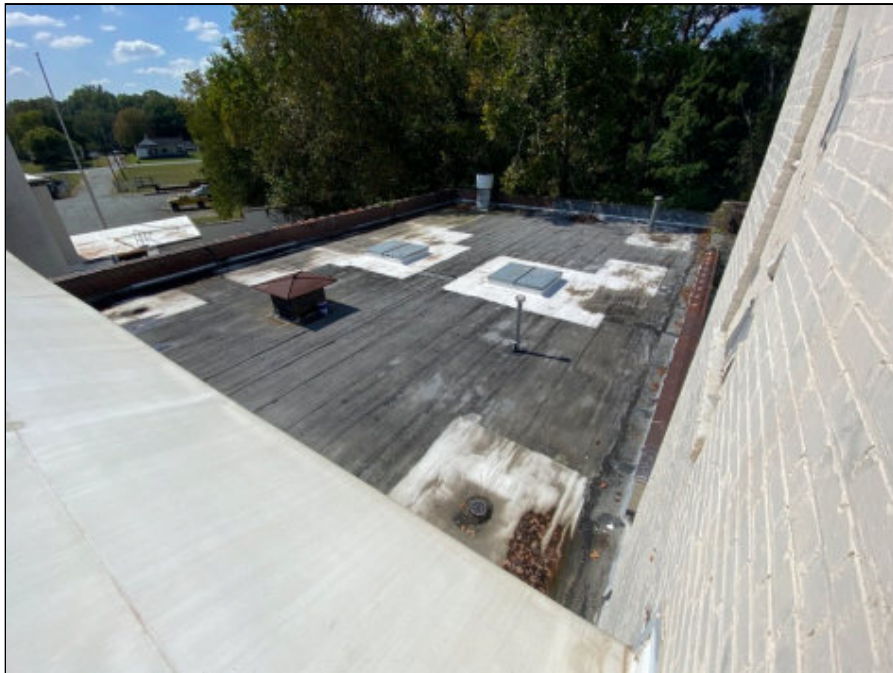
70 - Modified bitumen roof at west wing
