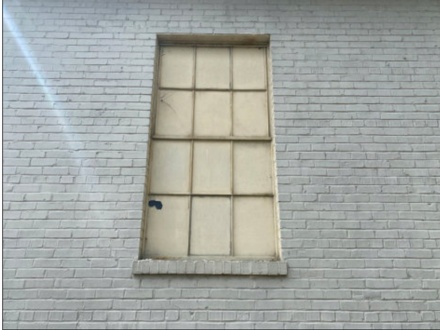
57 - Typical steel window (exterior view)
