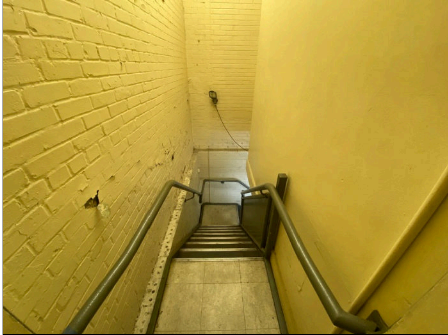
131 - Stairs (at upper level)
