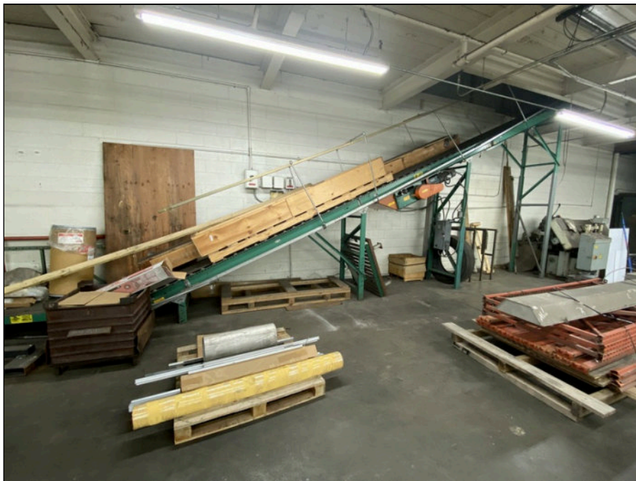
102 - Conveyor belt in plant area
