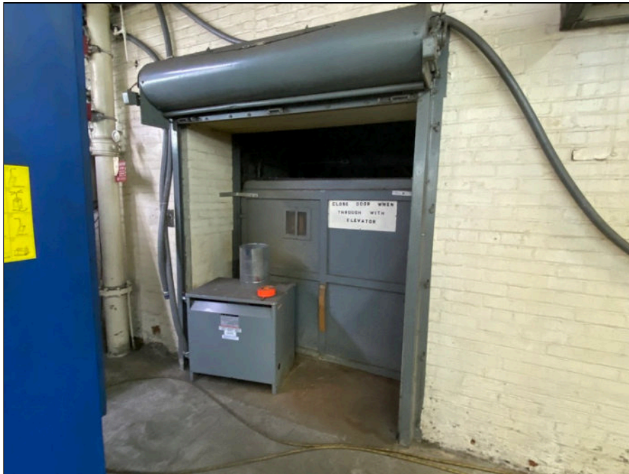
100 - Abandoned freight elevator
