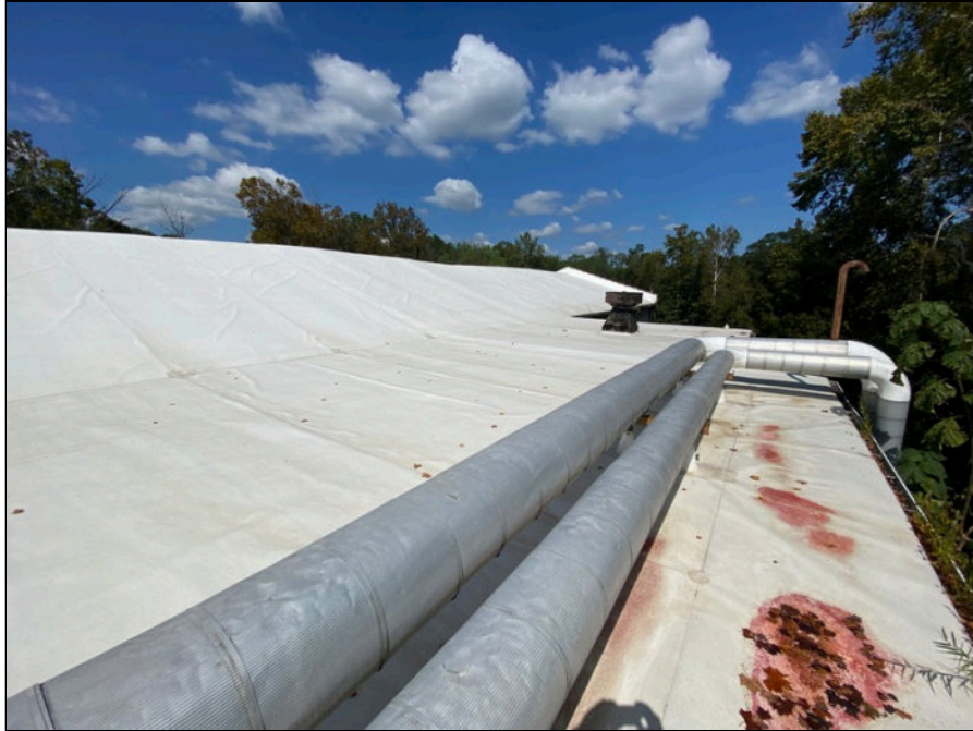
61 - View of roof
