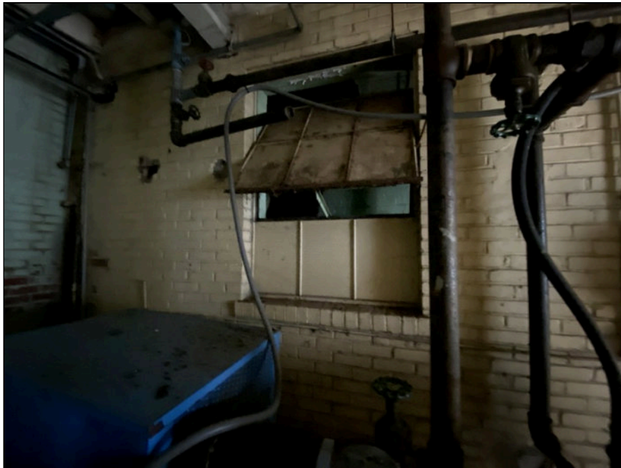
58 - Typical steel window (interior view)
