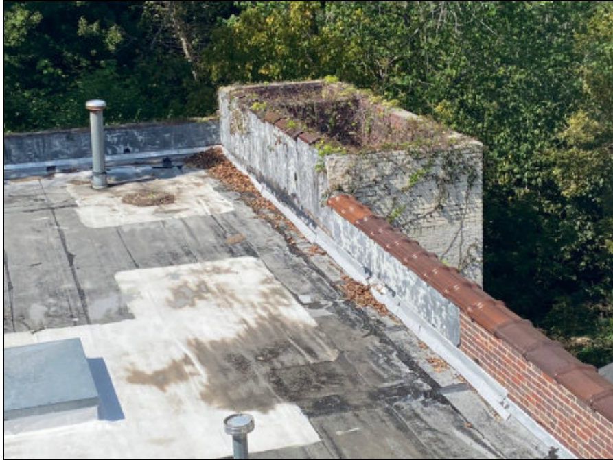
73 - Parapet at west wing
