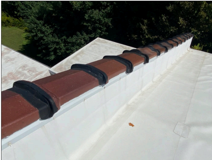
68 - Terra cotta coping at parapet
