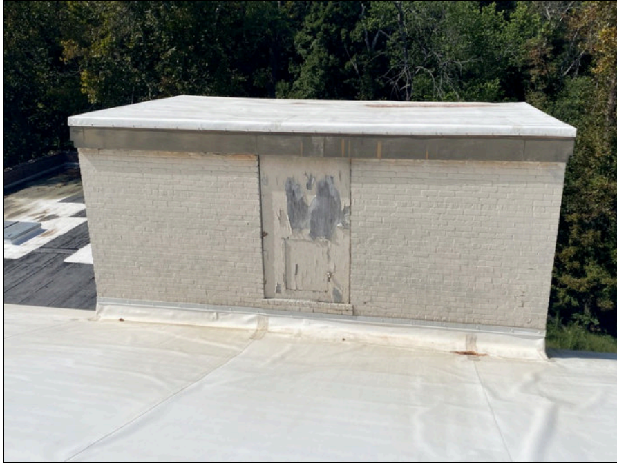
63 - Abandoned elevator penthouse
