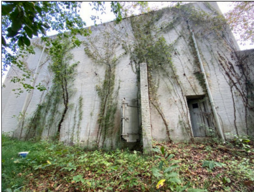
12 - West elevation (note ivy on walls)
