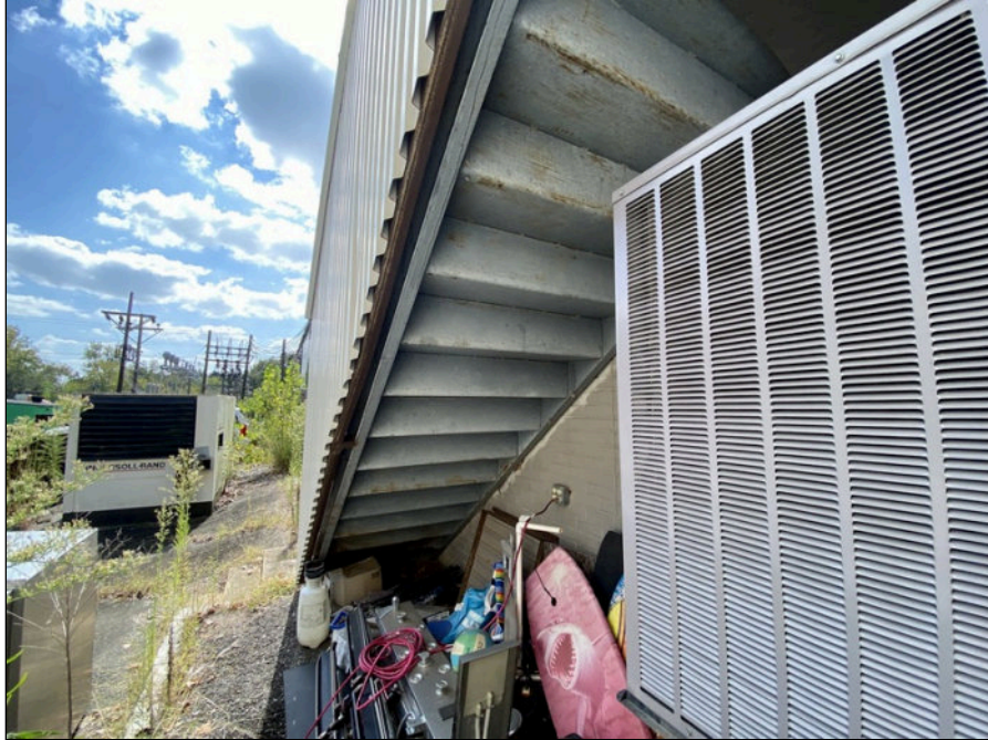
119 - Fire stairs at east side
