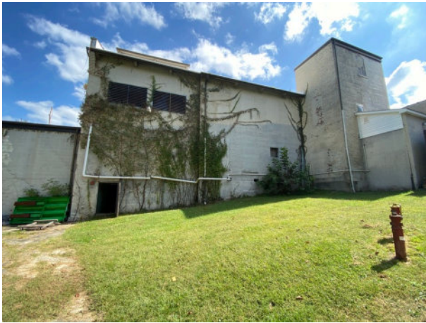
West elevation (note ivy on walls)
