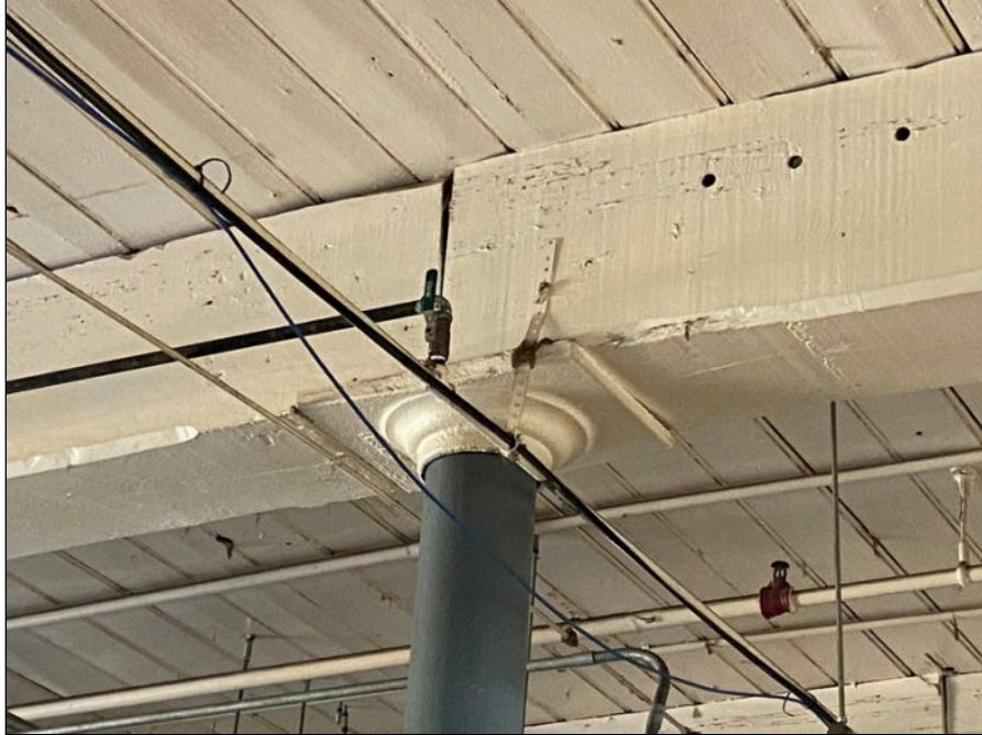
35 - View of typical interior wood beams
