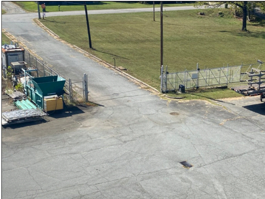
16 - View of entrance gate at Rush Street
