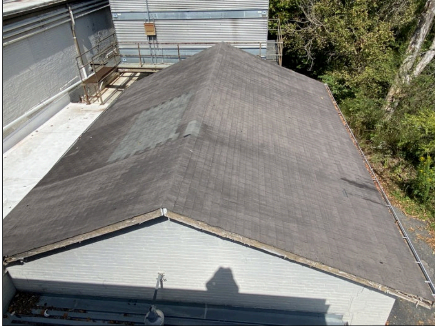
75 - Asphalt shingles at east side
