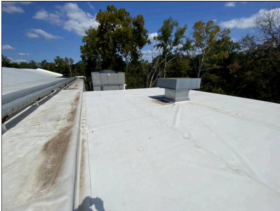
66 - View of roof
