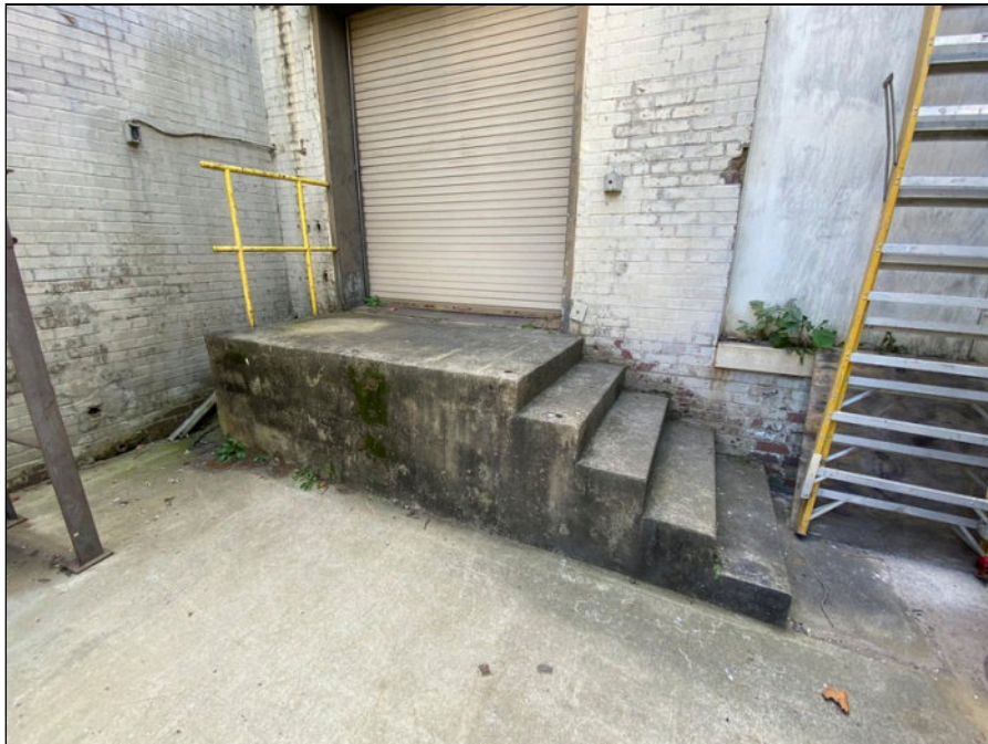
46 - Typical concrete steps at doorway
