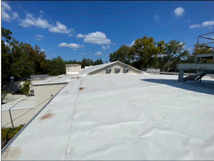
65 - View of roof
