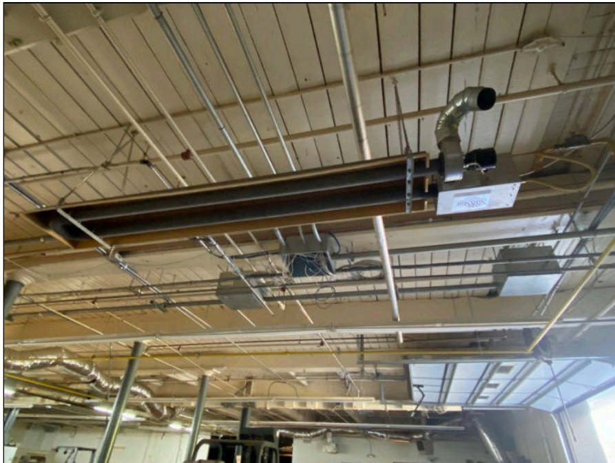
86 - Gas-fired unit heater
