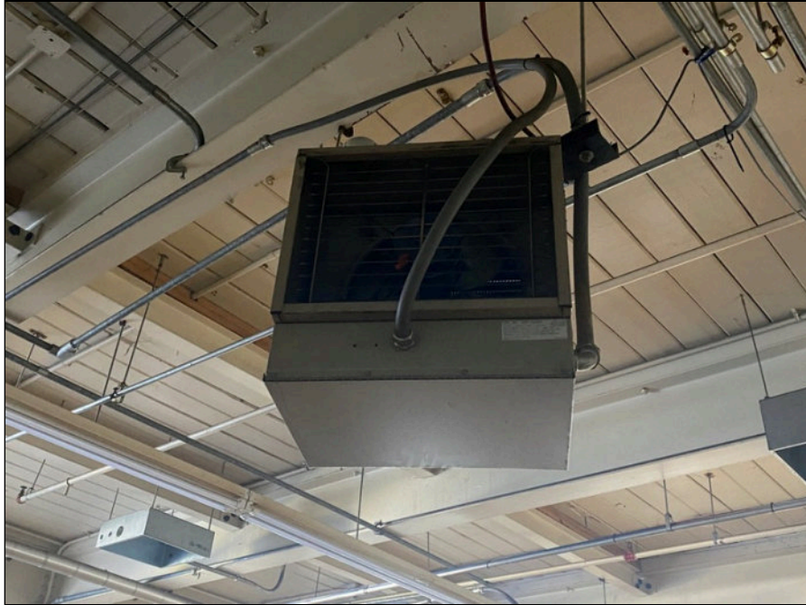
87 - Typical electric unit heater
