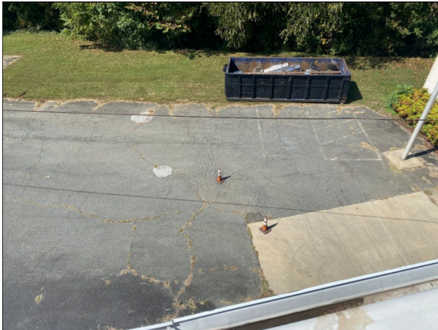
20 - Parking area at west side of building
