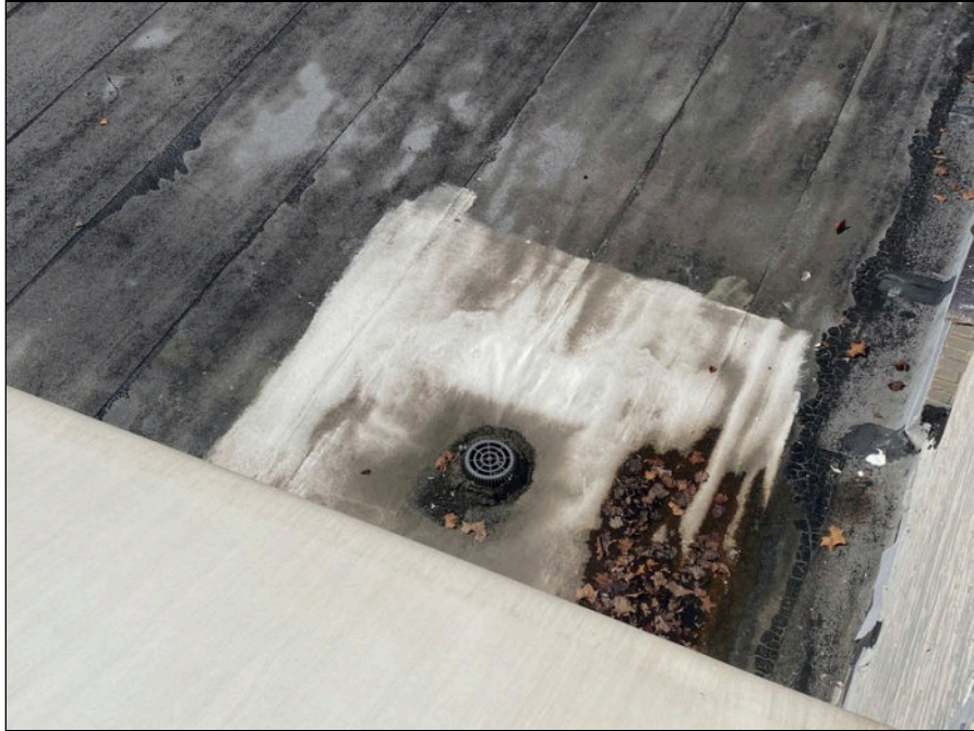
71 - Typical roof drain at west wing
