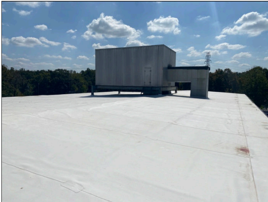
64 - View of roof
