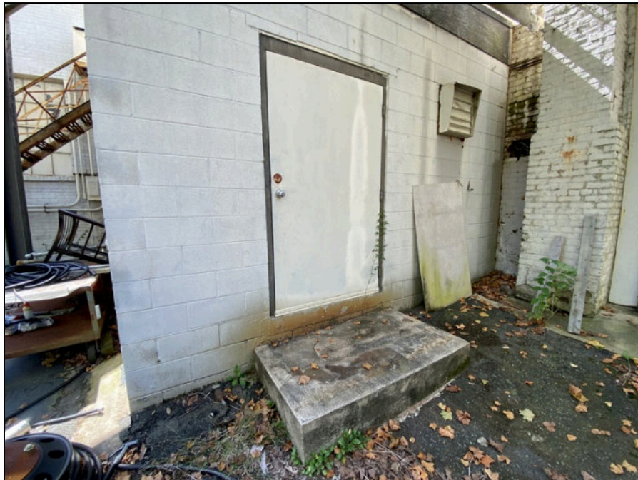
54 - Typical personnel door
