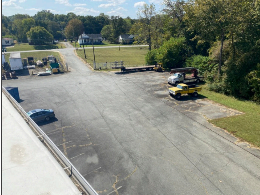
19 - Parking area at west side of building
