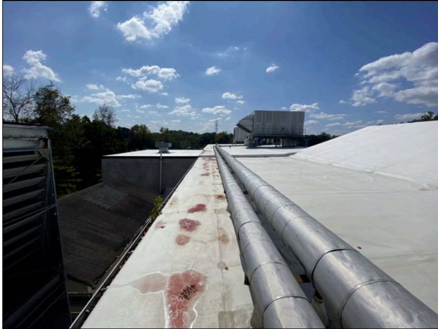
59 - View of roof
