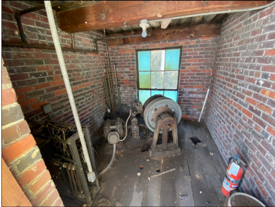
101 - Abandoned freight elevator penthouse
