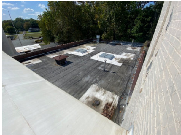
Modified bitumen roof at west wing
