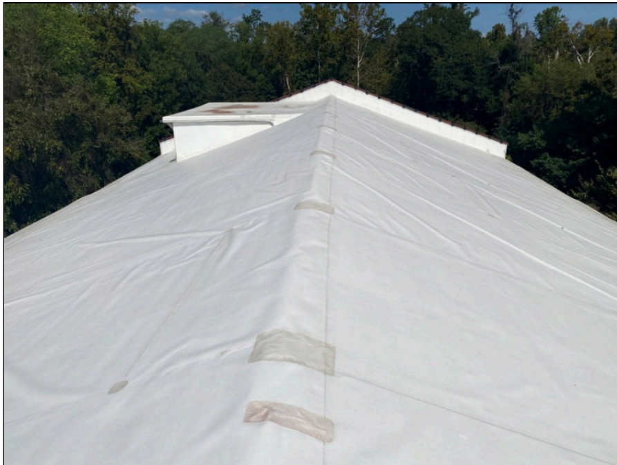
60 - View of roof
