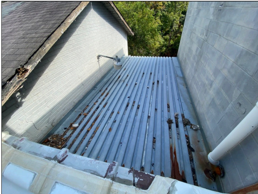
76 - Metal roofing at east side
