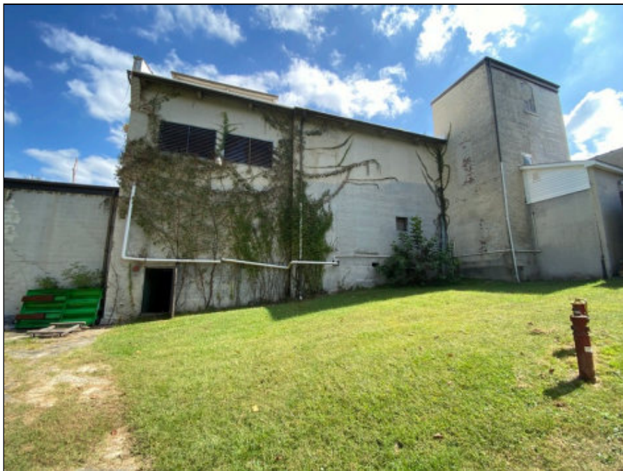
10 - West elevation (note ivy on walls)
