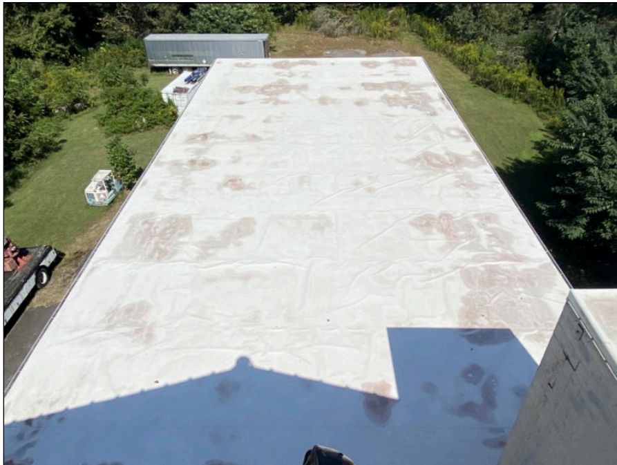
62 - View of roof at north end
